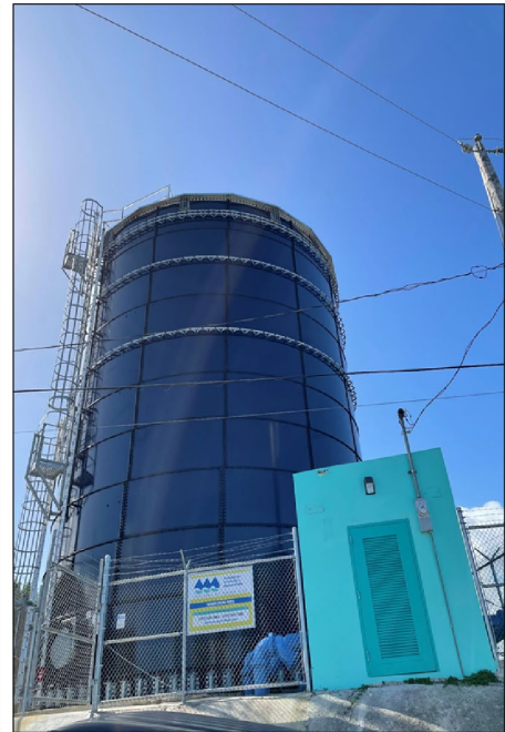
Largely repaired water tank observed in March in March 2022
