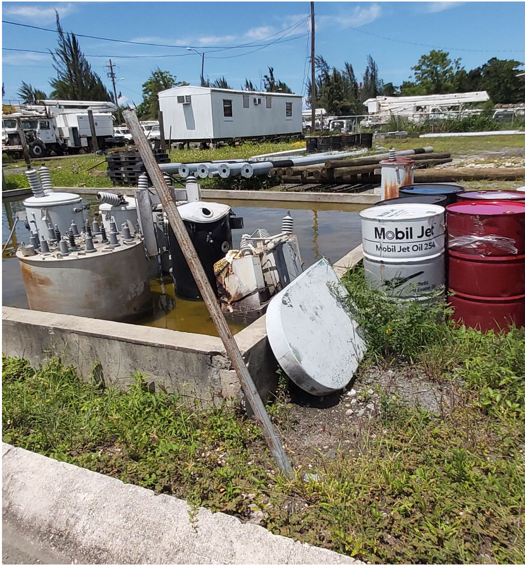
Palo Seco Transmission Warehouse Yard - Secondary Oil Containment about to overflow. Pre-LUMA System and Facility Conditions
