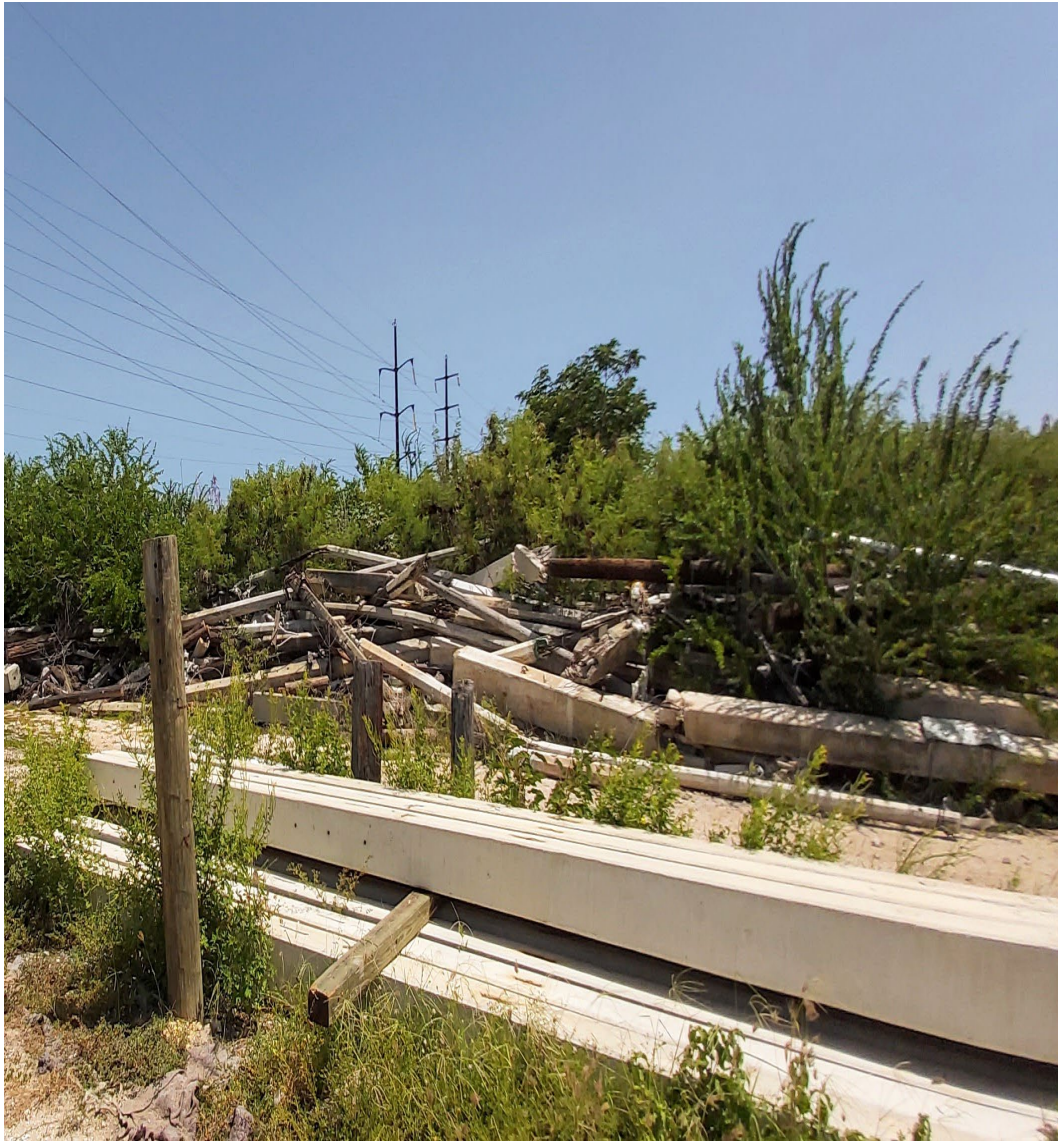
Ponce Secondary Yard - Scrap buried in the bush amongst 10' trees.
