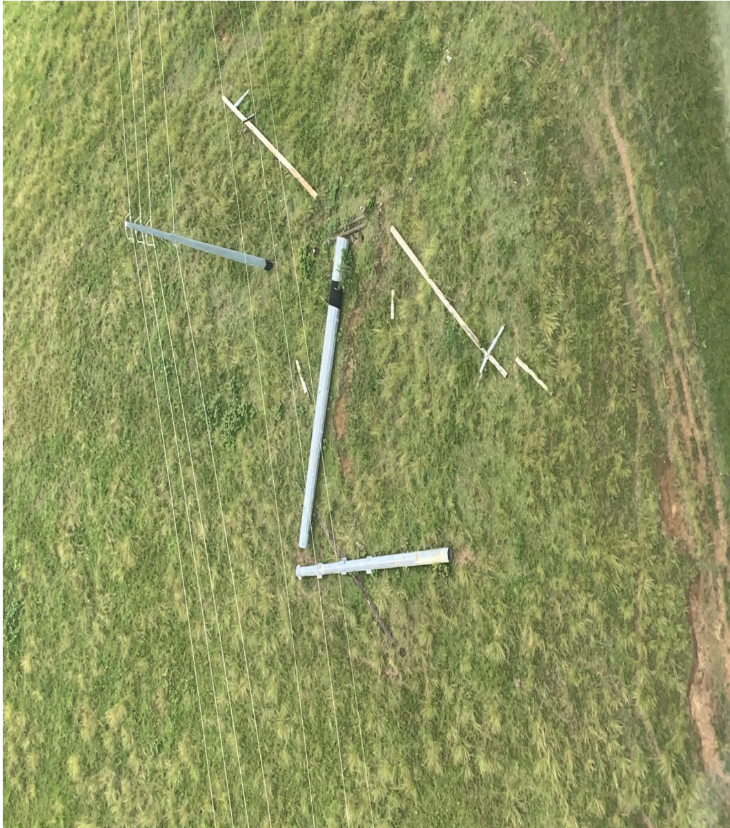
Failed Tx pole circuit.
