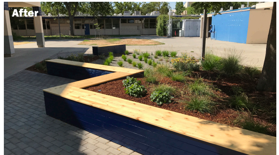
The new rain garden courtyard space features a rain garden and pervious paving system to collect, slow, and infiltrate stormwater. A series of strategically placed seatwalls direct pedestrian traffic around the newly transformed landscape area and create a beautiful space for students, teachers, and the overall community to enjoy.
