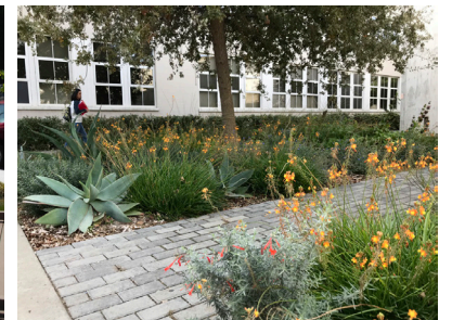
Pervious paver pathway
