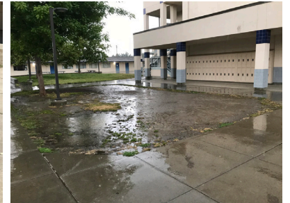
Existing site in storm event conditions
