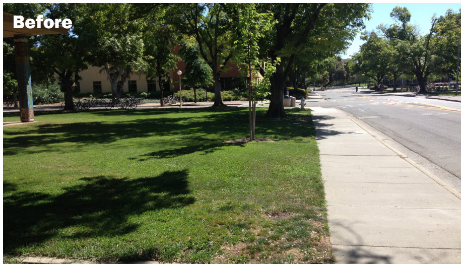
Prior to construction, this portion of California Avenue featured only water-thirsty turfgrass and street stormwater runoff was allowed to flow directly into an underground pipe system.
