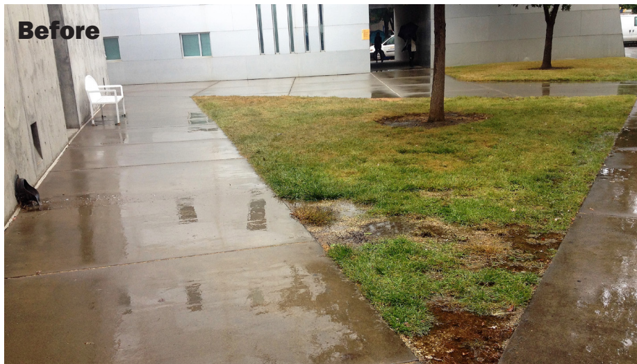
Before A building downspout at UC Davis' Social Sciences and Humanities Building directs stormwater runoff across a walkway and into an under-performing turf area. The California Student Leadership in Green Infrastructure immediately recognized the potential to transform the bland, non-functional space into a project with high environmental and placemaking value.
