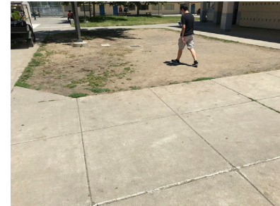
Existing site in dry conditions
