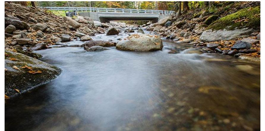
Roaring Brook culvert replacement: With a width of 35 feet, the new culvert – an open-bottom concrete box with a natural streambed – allows the stream to pass freely underneath, opening six miles of upstream habitat for fish and designed to withstand high water flows.
