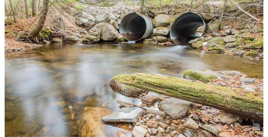
Roaring Brook culvert prior to replacement. At lower flows this culvert outlet was perched above the water surface, creating a barrier to the movement of fish. The stream was constricted by the pipes' combined span of 12 feet, which caused debris build-up and localized flooding.
