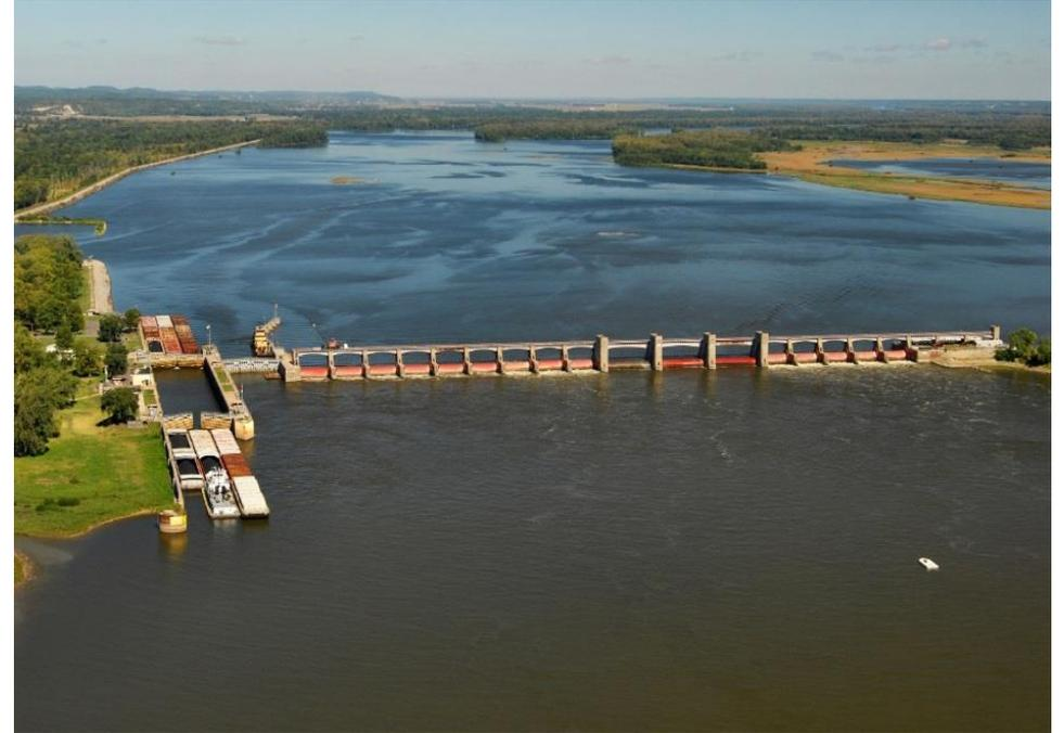
Lock extensions from 600' to 1200' will increase efficiency at the 7 lock improvement sites by eliminating the need double locking (as shown in picture) which is standard practice at all but two locks on the 37 lock system of the UMR. Disintegrating concrete and mechanical systems will be rehabilitated or replaced as the lock is lengthened.
